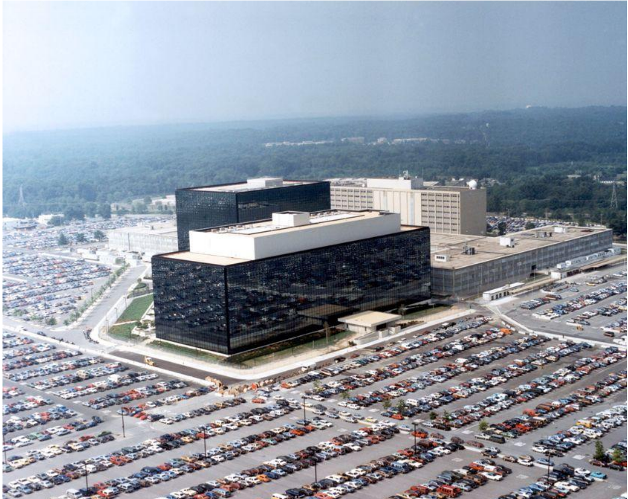
The OPS2A and OPS2B buildings at NSA'S headquarters in Fort Meade, MD. Their exterior glass is laced with copper to prevent signals from leaking; classical music plays to deter eavesdropping.
